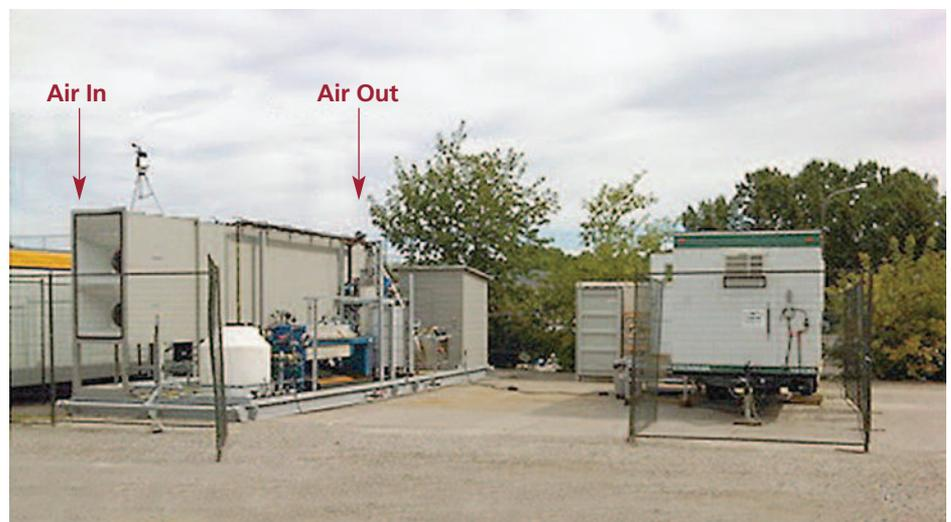
Carbon Engineering’s air capture prototype uses an oxy-fuel natural gas kiln to drive the CO<sub>2</sub> out of the solid calcite.
